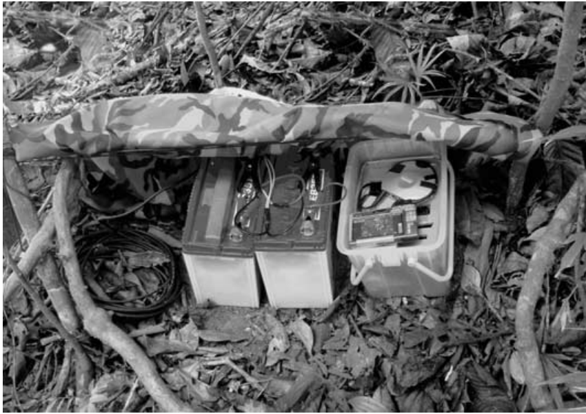
Fig. 2. Field installation of digital video surveillance system covered by camouflaged waterproof material. Plastic box contains video recorder, adaptor and cigarette lighter connectors to connect to the deep cycle batteries.
